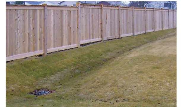
Rear-yard swales direct flows to a catch basin in this image. Rear-yard catch basins and swales shouldn't be covered or filled in with backyard sheds, fences or other structures, and rear-yard catch basins should be kept clear to reduce backyard flooding.
